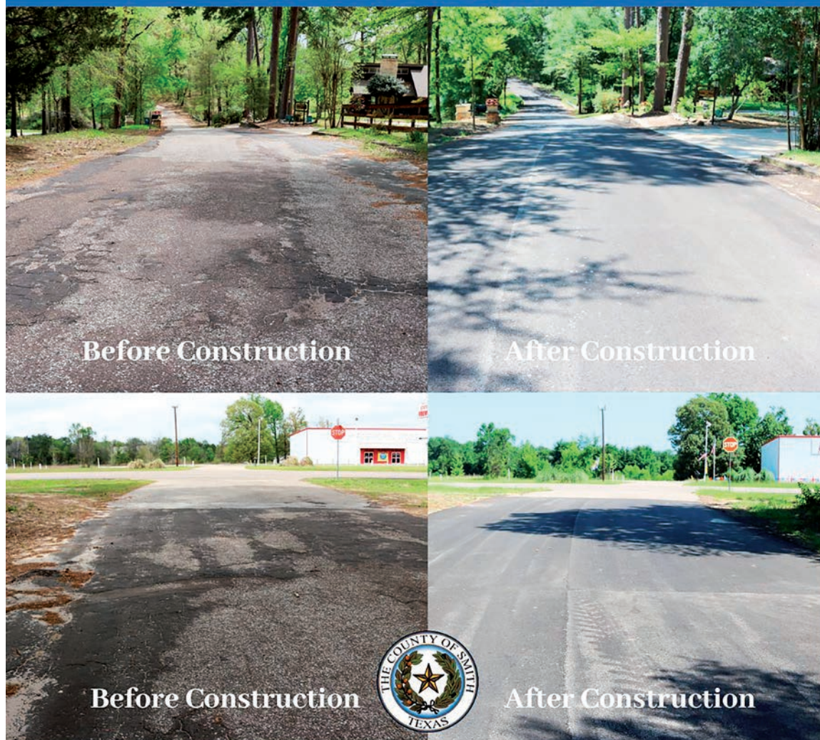
County Road 2212, also known as Surrey Trail, is shown in before and after photos.
