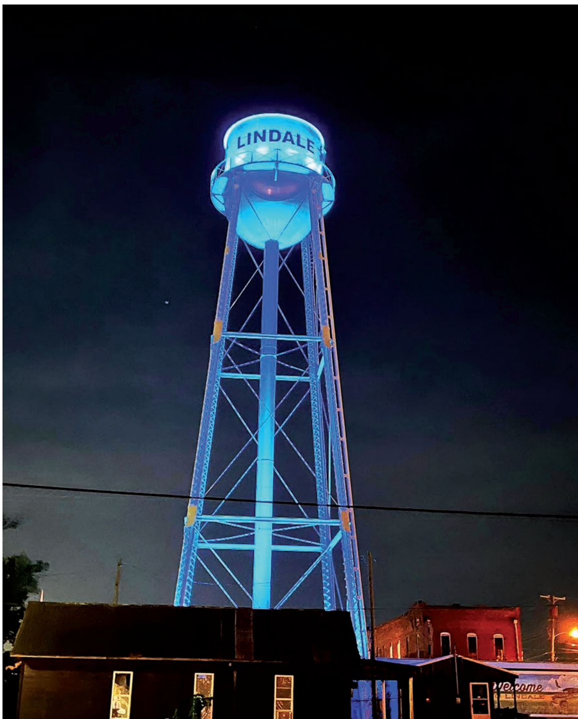
After a dedication ceremony on Wednesday May 3, city officials flipped a switch and the historic downtown water tower became a brilliant, blue beacon in the night.
